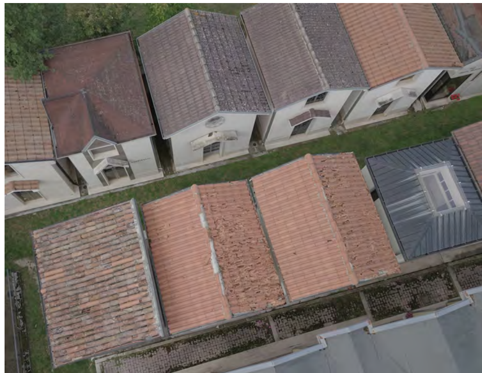
Figure 1. An example of roof tiles characterized by different shape, dimensions, colors and integrity.
