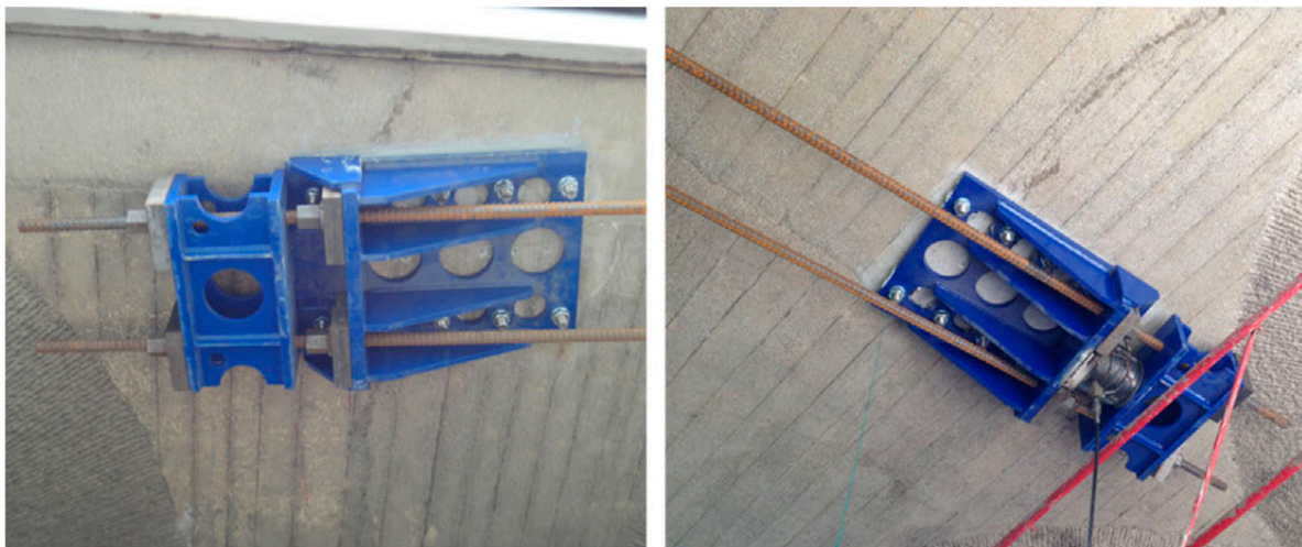
Figure 22. Passive (left) and active (right) anchorages.
