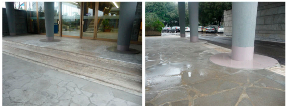
Figure 12. Visual impact of the intervention at the end of the work.
