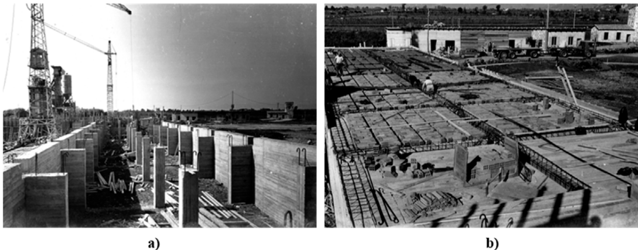
Figure 6. Archive photos of the Reinforced Concrete (RC) box at the basement: (a) before and (b) after the realization of the slab (note that the clay blocks, with which the slab is made, are clearly visible).
