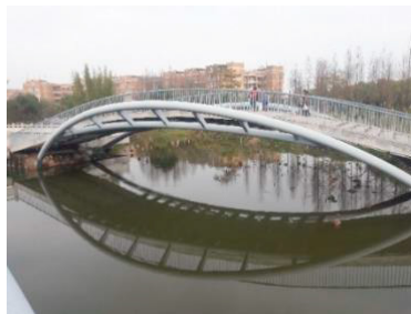
Fig. 1. The butterfly-arch stress-ribbon pedestrian bridge in Fuzhou University, Fuzhou, Fujian, China.
