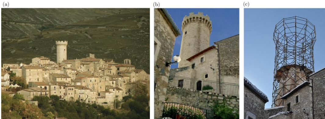
Fig. 1. (a) Location of the Medici tower in the landscape and within the town core; (b) architectonic configuration of the tower before the 2009 L'Aquila earthquake; (c) reproduction of the tower's original profile through scaffolding placed after the collapse in 2009.
