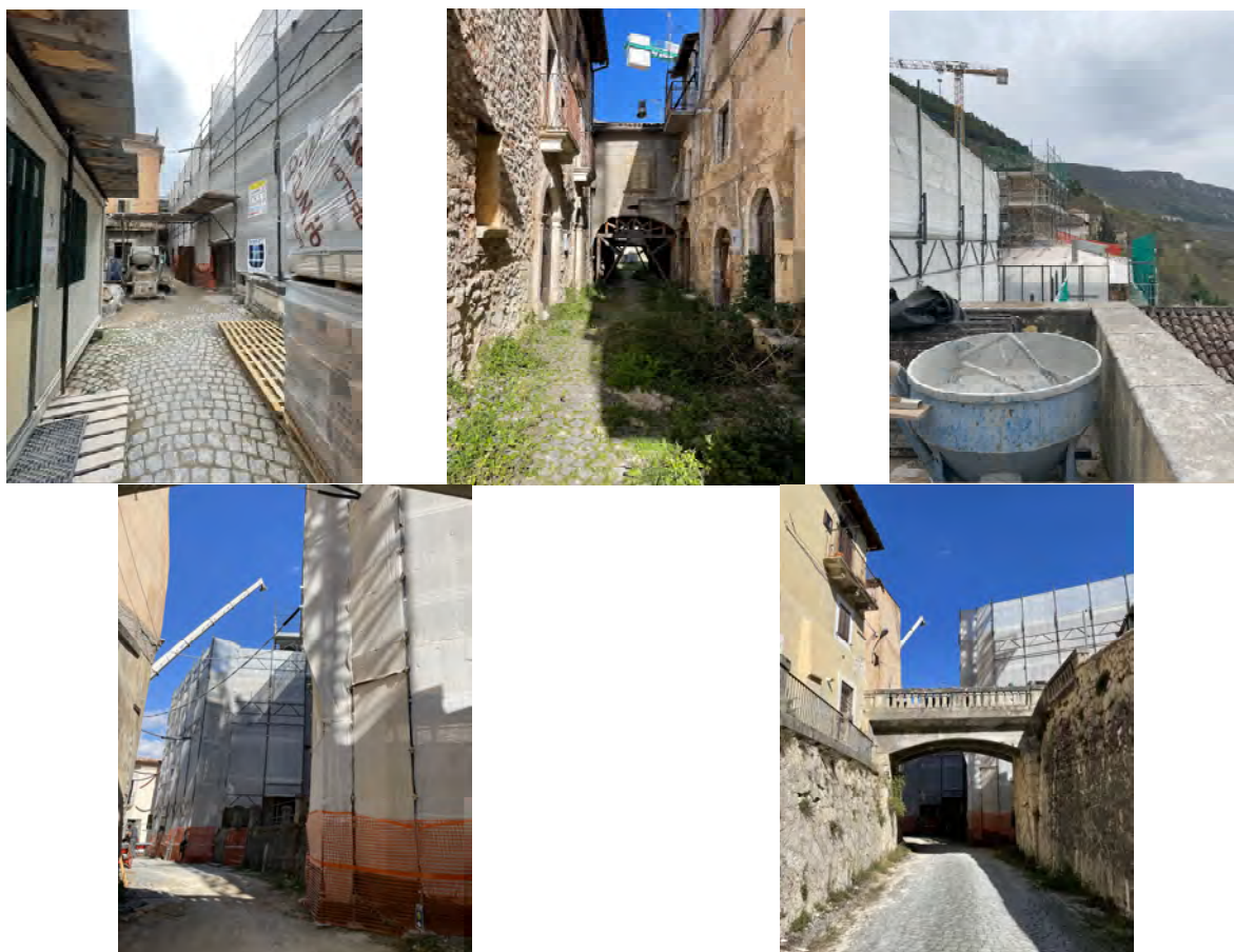
Figure 5. Construction site views of Palazzo Lazzaro.
