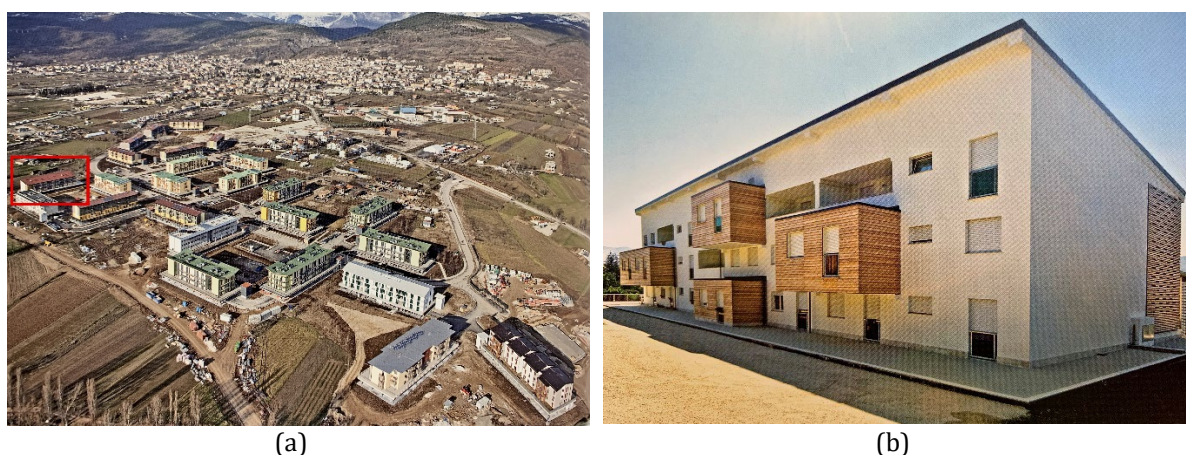
Figure 2. Building B2. (a) Territorial framework. (b) View of the building.
