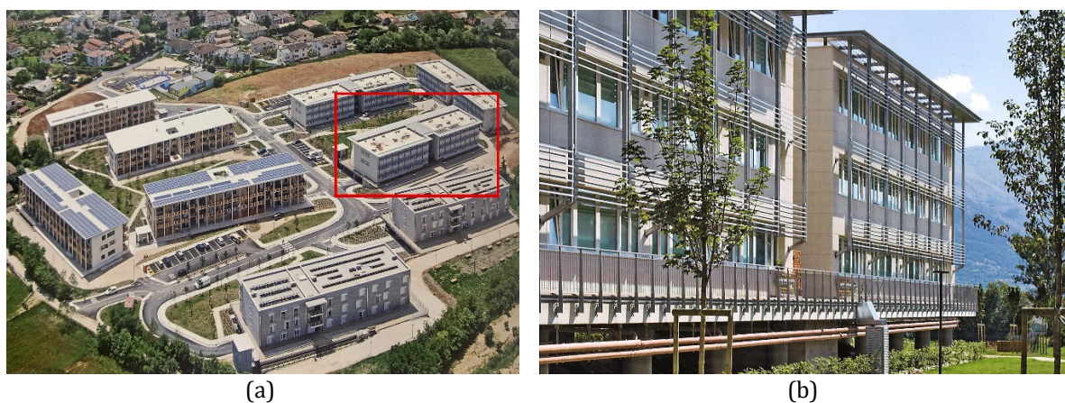
Figure 1. Building B1. (a) Territorial framework. (b) View of the building.
