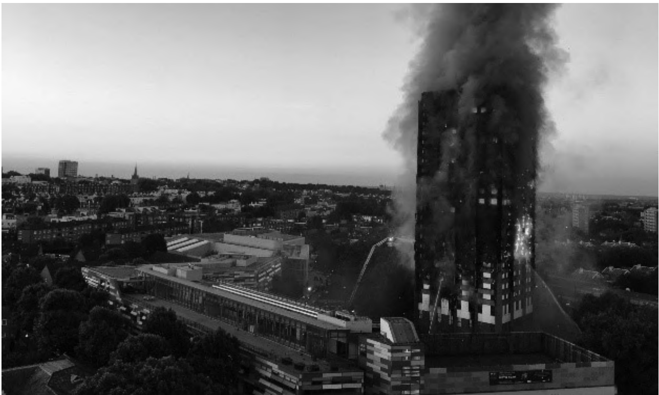
Figure 5. Fire at the Grenfell tower, London, 2017
