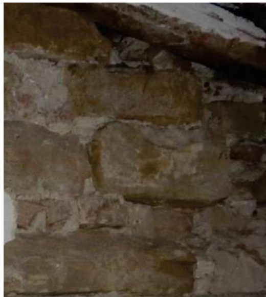
(b) Tuff masonry with scattered clay units.
