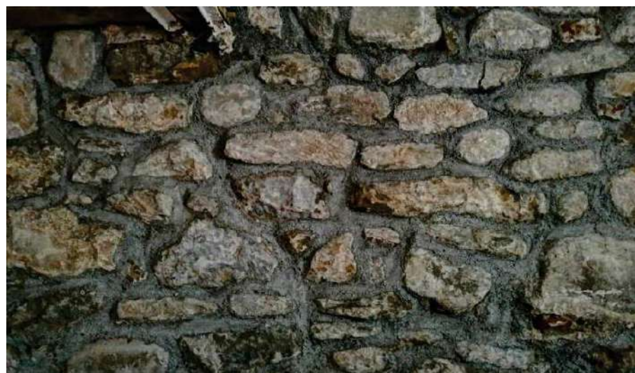
Figure 3.14. Texture of the masonry.
