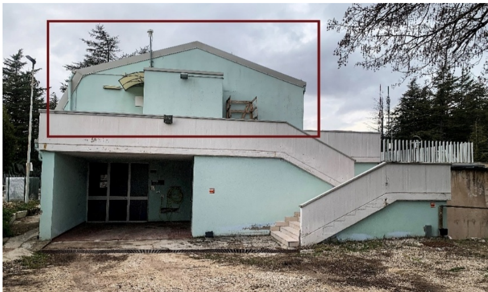
Figure 1. Front view of the sample building.
