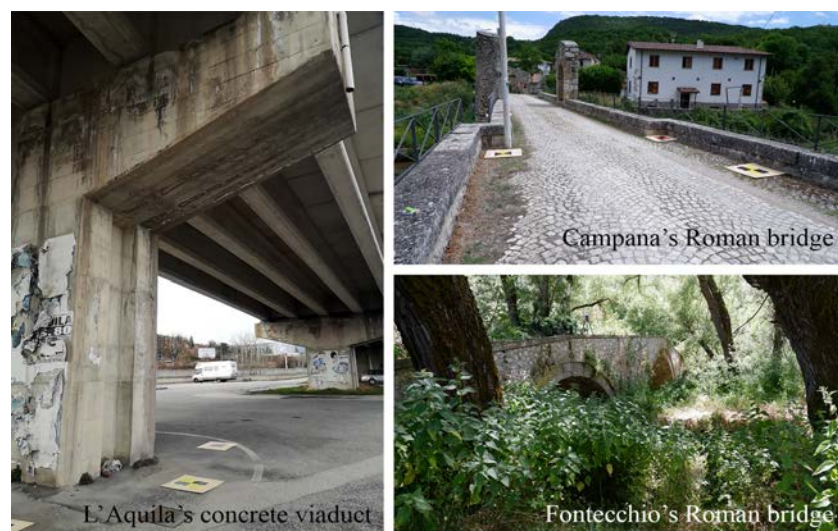
Figure 1. Case studies: concrete pillar of a viaduct in the city of L'Aquila, Roman bridge in the rural area of Campana, and the Roman bridge in the vegetated area of Fontecchio.
