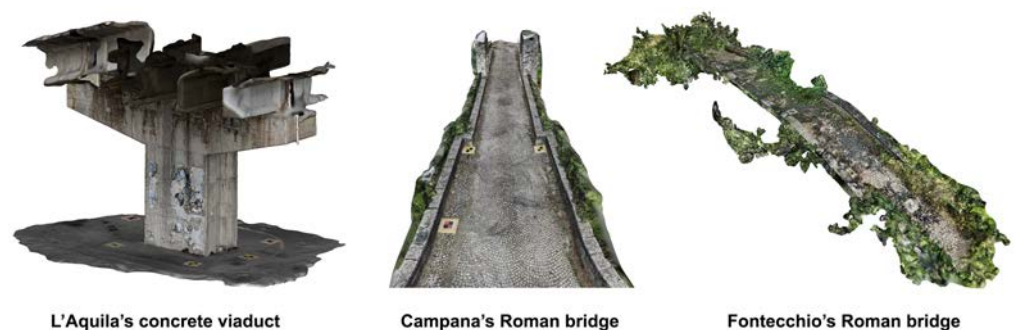
Figure 11. The 3D models of the viaduct in L'Aquila and the Roman bridges in Campana and Fontecchio acquired using mobile phones equipped with the viDoc RTK Rover and processed with PIX4Dmatic.
