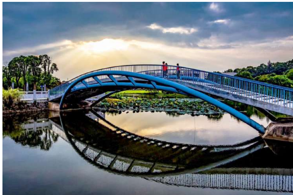
Figure 6.1. The butterfly-arch stress-ribbon pedestrian bridge in Fuzhou University, Fuzhou, Fujian, China.
