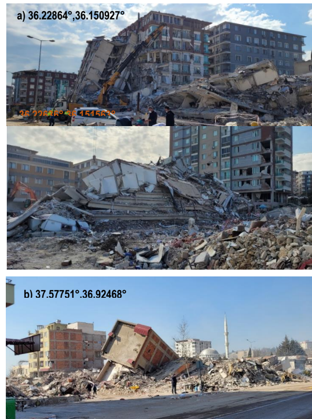
Fig. 2. Damage photos from the region. a) Images from Central Antakya - above alluvium. b) Images from Kahramanmaras city center, a city settled on alluviums, buildings around stream bed.
