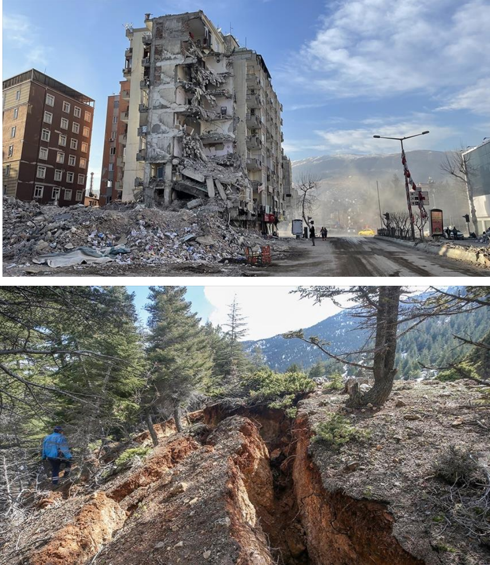
Figure 5. Observed damage in Göksun city (Photos from Anadolu Ajans, https://www.aa.com.tr/tr/asrin-felaketi/kahramanmarasin-Göksun-ilcesinde-5-1-buyuklugunde-deprem-/2824289 , https://www.aa.com.tr/tr/asrin-felaketi/Göksunda-deprem-nedeniyle-derin-yariklar-olustu/2837685 ).
