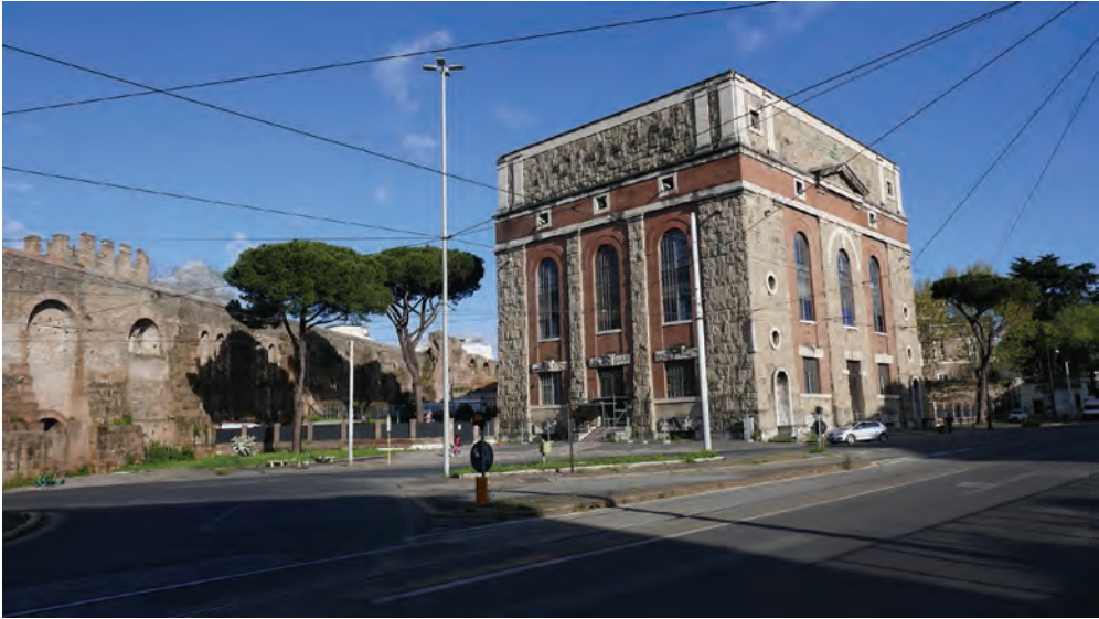
Figure 2.3.16 The water reservoir on via Eleniana standing out against the city walls, here coinciding with the Claudian aqueduct, Rome.
