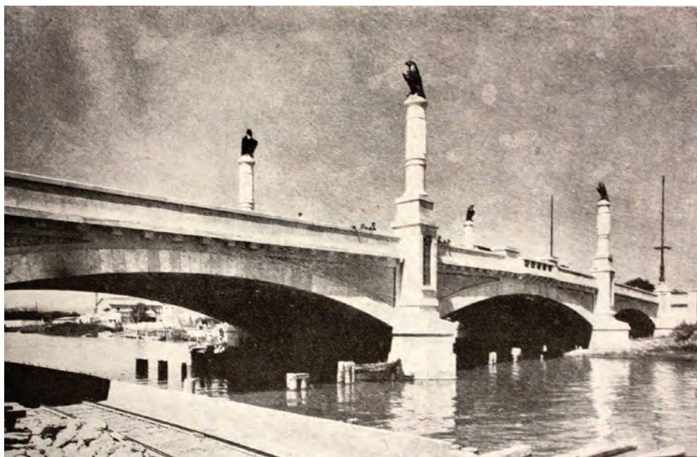
Figure 2.3.5 Pescara, Ponte Littorio over the river Pescara: photo just after work was completed.
