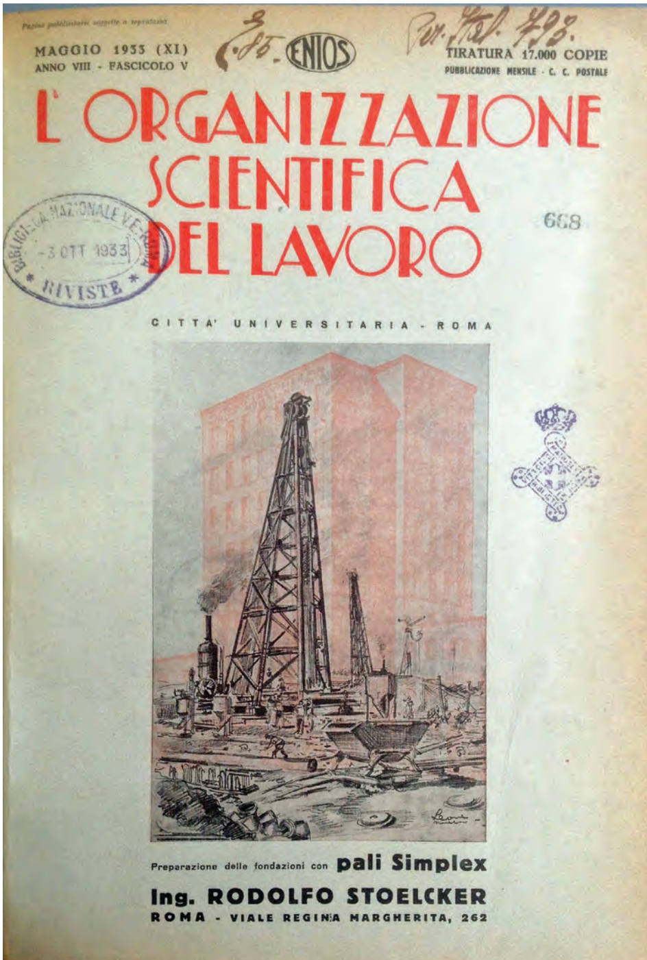
Figure 2.3.19 Pile driving structure used by Stoelcker for the construction site of the University City of Rome.
