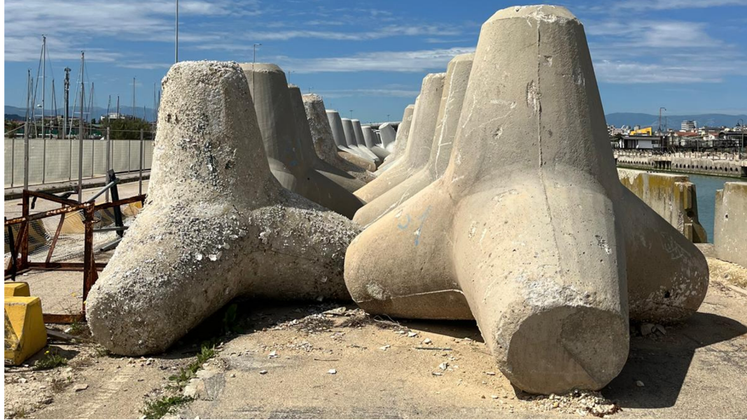
Figure 3.10. Tetrapod concrete armor unit (Photo of the author)
