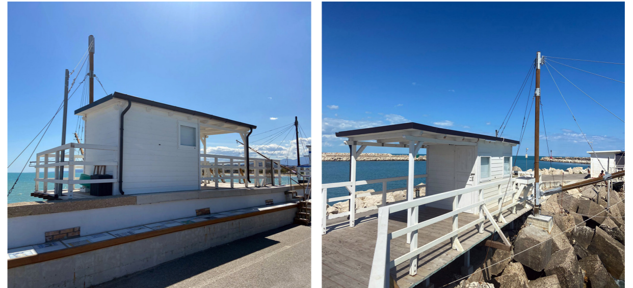
Fig. 9 - Completion of the caliscendi with the pier and access ladder (Marchionni C. 2022).
