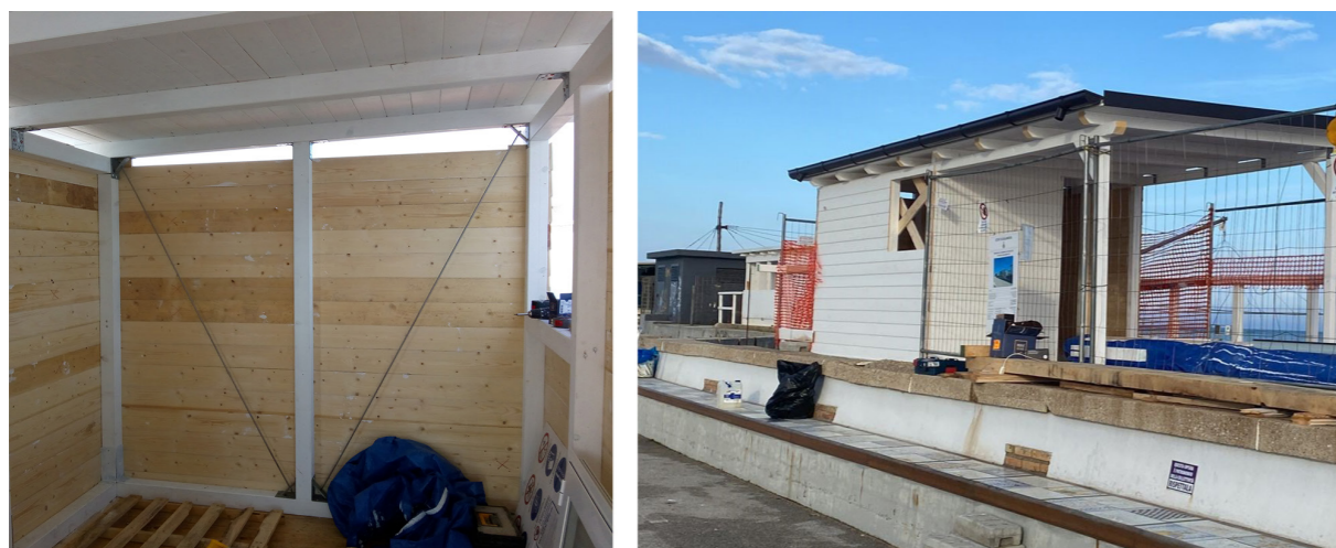
Fig. 8 - Construction of perimeter walls and finishing elements (Marchionni C. 2022).
