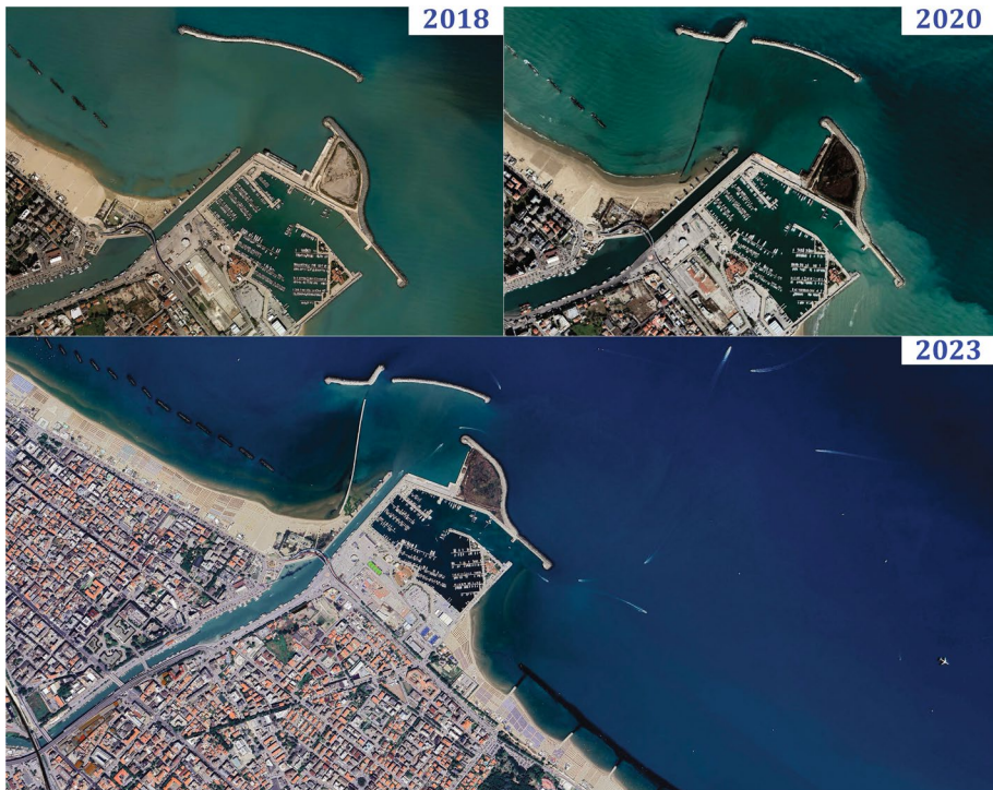
Fig. 5 Achieved steps toward the completion of the Pescara River mouth deviation. Comparison over the years. Source Google Earth
