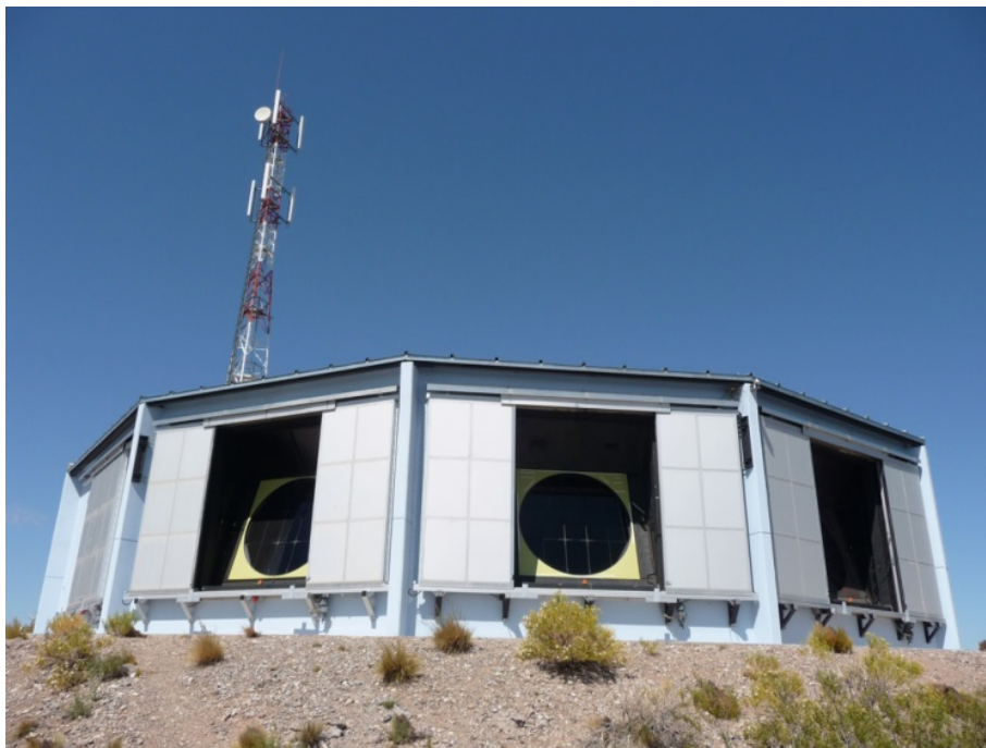
Figure 3.4: FD building at Los Leones. From [35].
