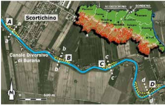
Figure 1. Aerial view of the damaged bank stretch and location of the investigated areas.
