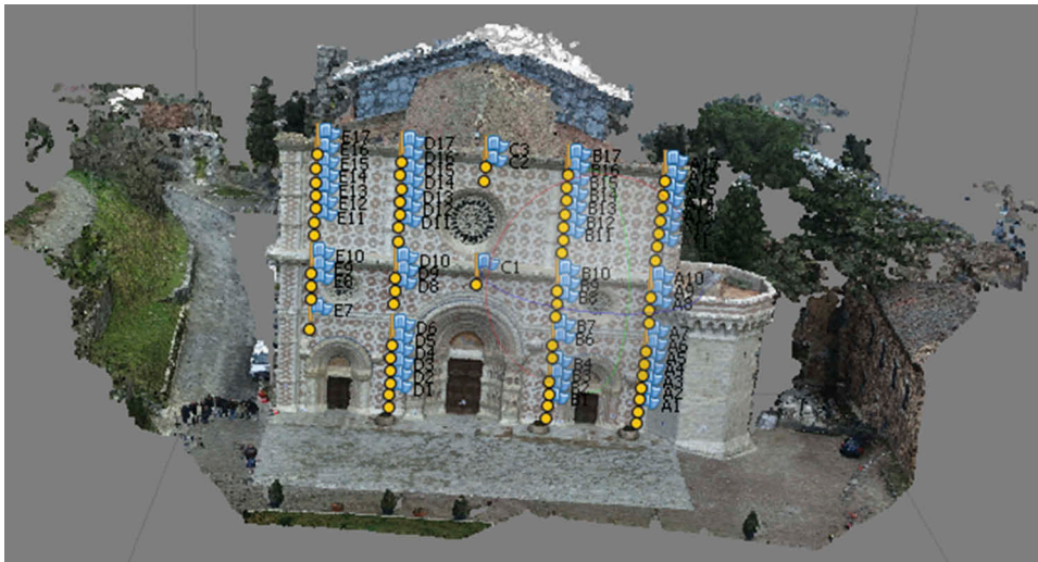
Figure 13. Point cloud of the Basilica di Collemaggio produced by Agisoft Photoscan following a UAV survey and ground control points obtained with a total station.
