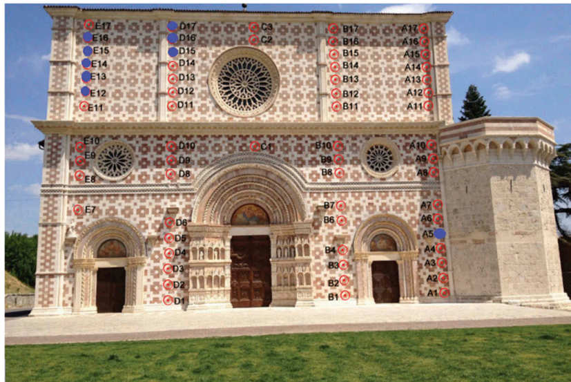
Figure 12. Measured points on the façade of the Basilica di Collemaggio, in blue unused points, suspect outliers.
