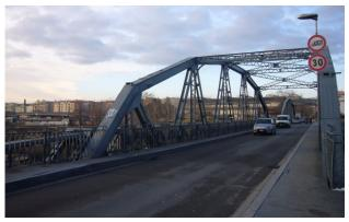
Figure 12. Industry Bridge transformed using iron elements of Alari Bridge
