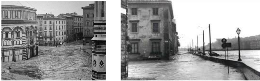
Figure 3. Two images about the flood of Florence (1966).
