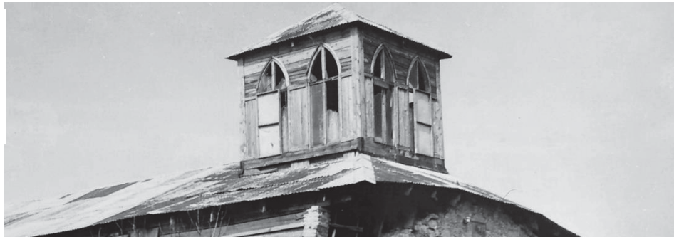
Fig. 3.36 The church of Sant'Orante with the provisional structure in timber ("lantern") (1960, ASGCRReg_Az)
