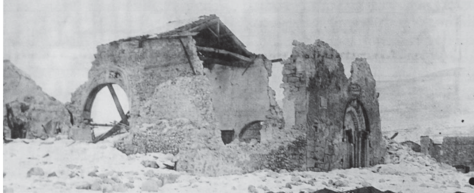
Fig. 3.34 Church of Sant'Orante after the earthquake of 1915.
