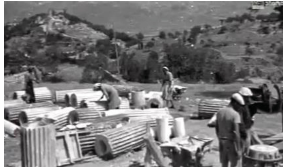
Fig. 3.68 – Fig. 3.69 Workers during the deassemblation of the elements and the cataloguing.
