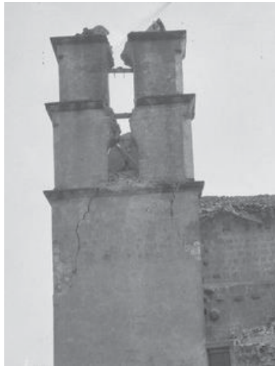
Fig. 4.26 – Fig. 4.27 left and right Picture of Mission Santa Barbara after the earthquake of 1925. Detail of the bell tower (USCS).
