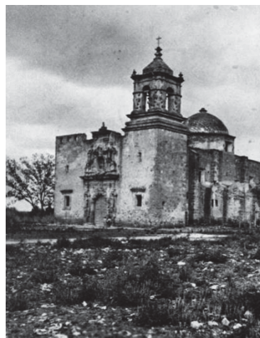
Fig. 4.35 - left Picture of the façade of the church, after the collapses of the interior (TSA)
