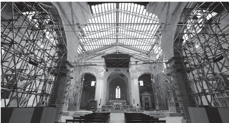
Fig. 5.20 Interior of Collemaggio with the provisional structures after the earthquake, view from the nave.
