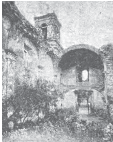
Fig. 4.41 - left Interior of the church after the collapse (Ford Powell and Carson)
