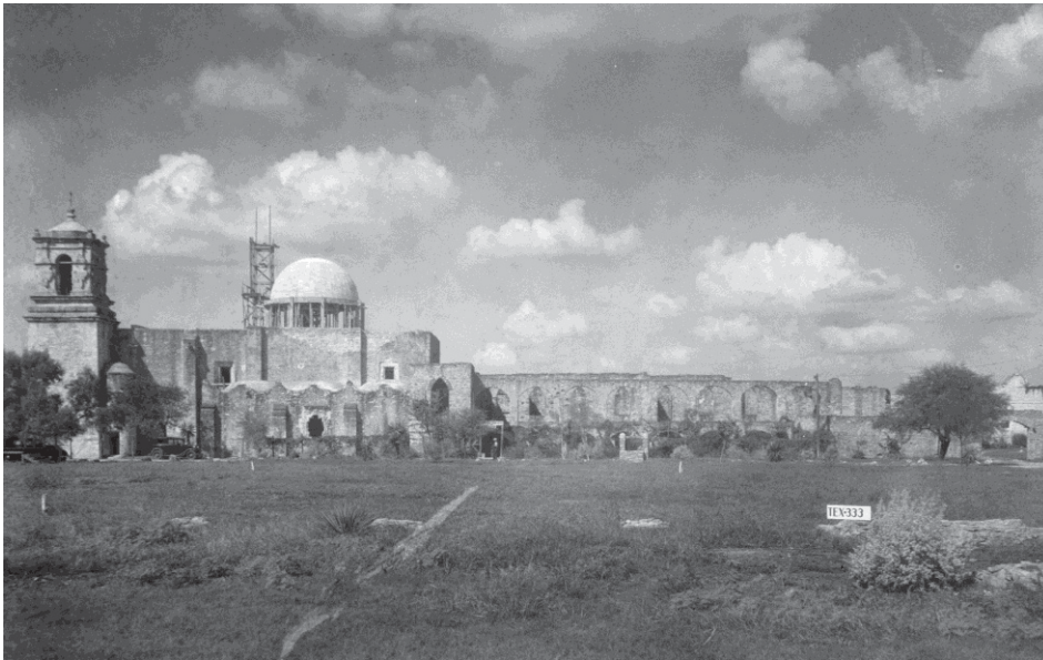
Fig. 4.54 Lateral view during the reconstruction of the dome (1936) (HABS)
