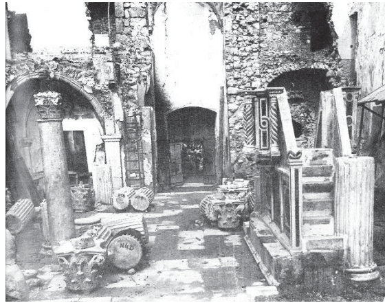
Fig. 3.70 View of the main gate of the church after the liberation of the interior from the ruins.
