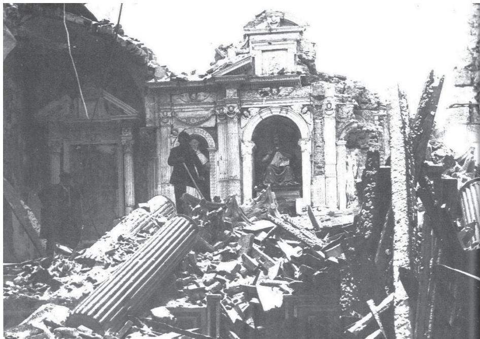
Fig. 3.65 Interior of the church of San Pietro in Albe during the first phase of liberation from the ruins.
