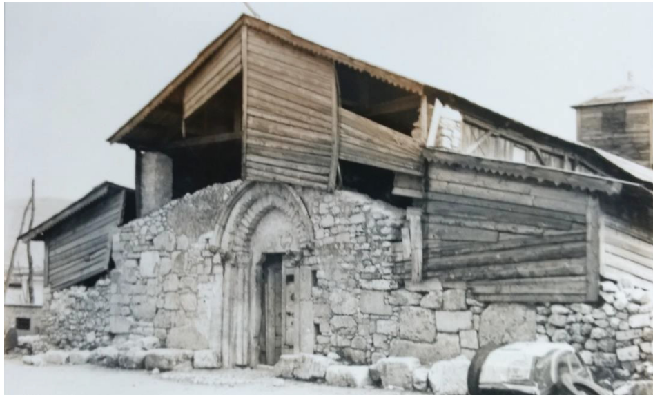
Fig. 3.35 The church with the provisional structure in timber (front) (1960, (ASGCRReg_Az)
