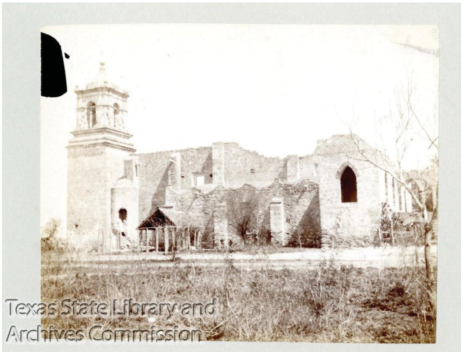
Fig. 4.38 Picture of the mission of San Jose after the collapse of the dome. (TSA)
