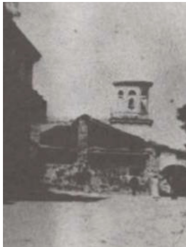
Fig. 4.7 (left). The San Juan mission after the earthquake of 1906. With the collapse of the convento's walls (SJHS).
