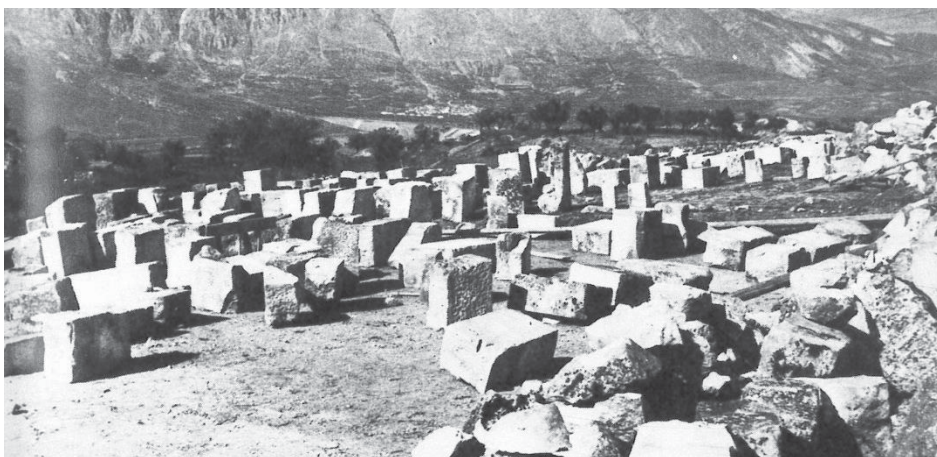
Fig. 3.73 The disassembled elements of the church
