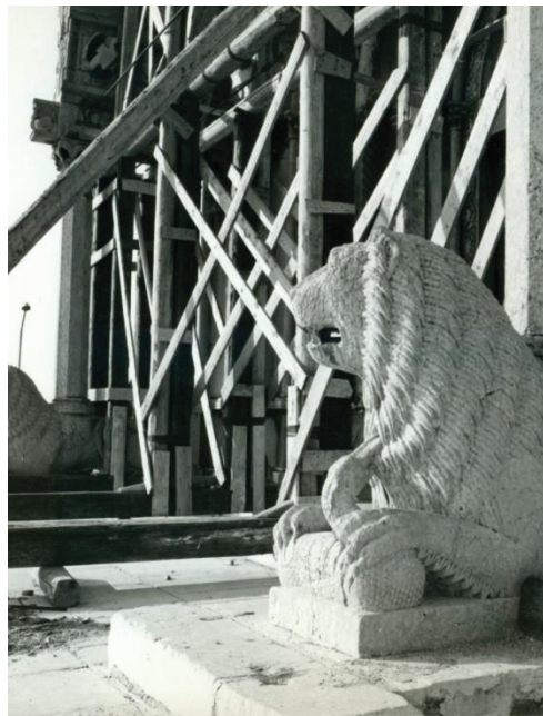
Fig. 1.3 - left Church of Santa Maria Maggiore in Tuscania after the earthquake of 1971 (A_4|9).
