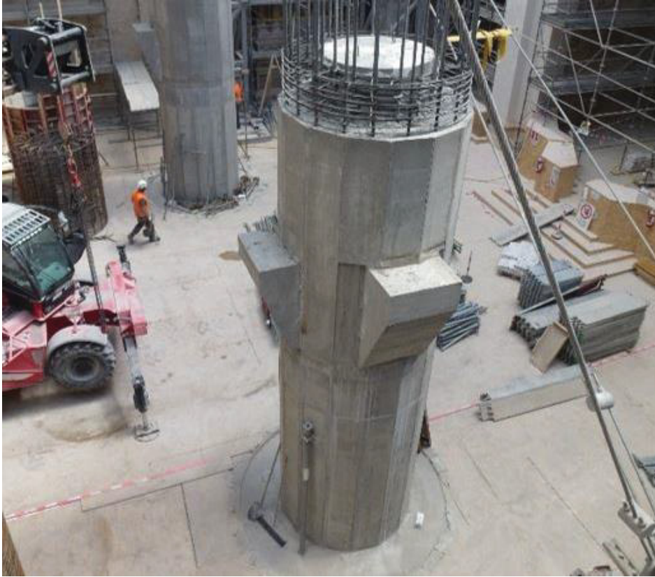
Fig. 6.2 The new pillar in reinforced concrete, realized in the reconstructed area.
