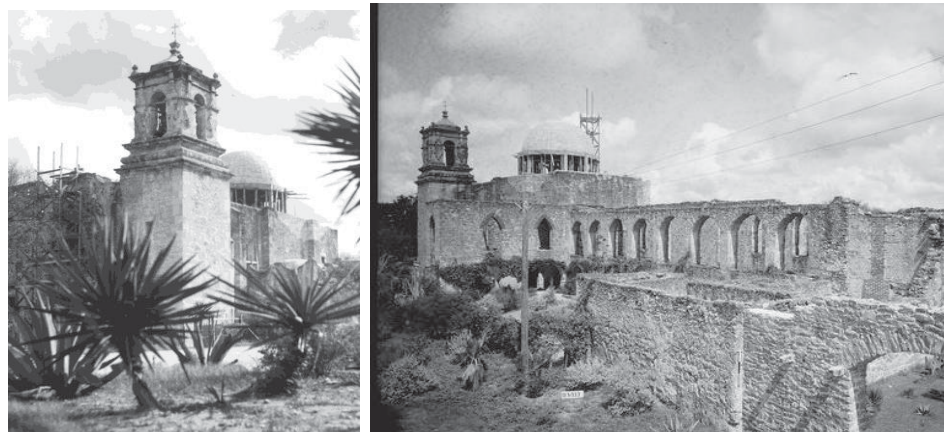
Fig. 4.52 - left Scaffolding covers the entrance to the church while a waterproofing compound is applied to the carved stone façade, (November 1935) (UTSA)
