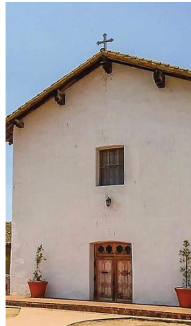
Fig. 5.6 – left Mission San Miguel Archangel in 1936. Front Façade (HABS).
