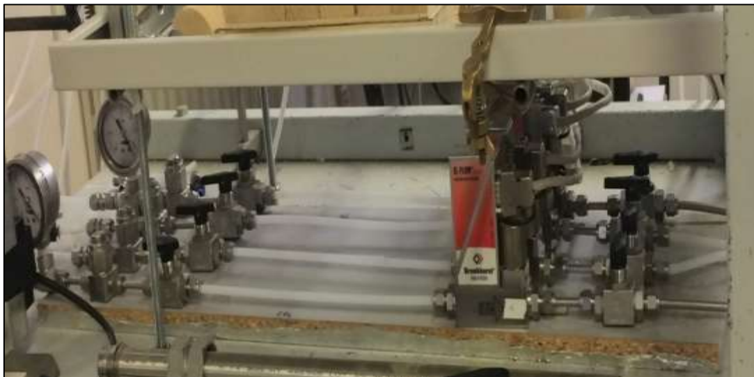
Figure 3.14: Gases supply lines
