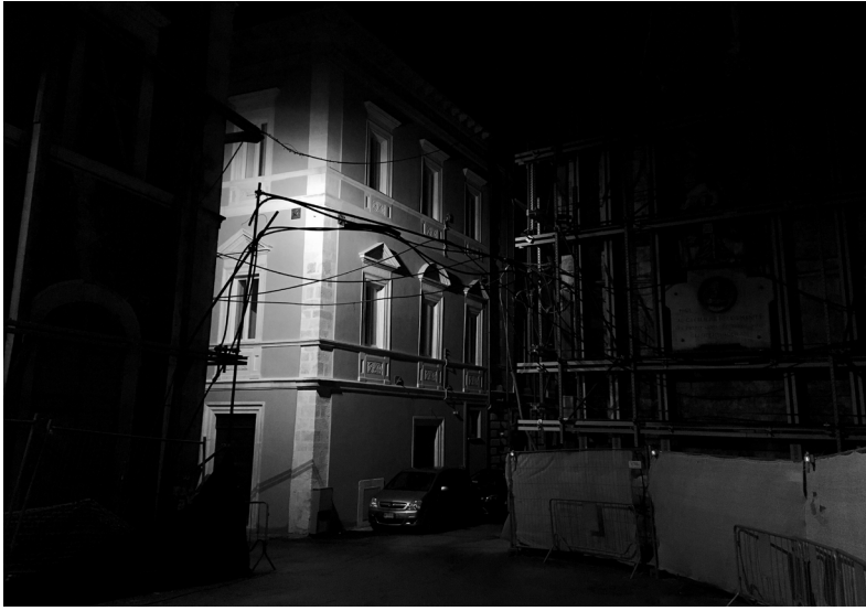
Figure 14.4 Building site at night. Photo: Fatima Marchini.
