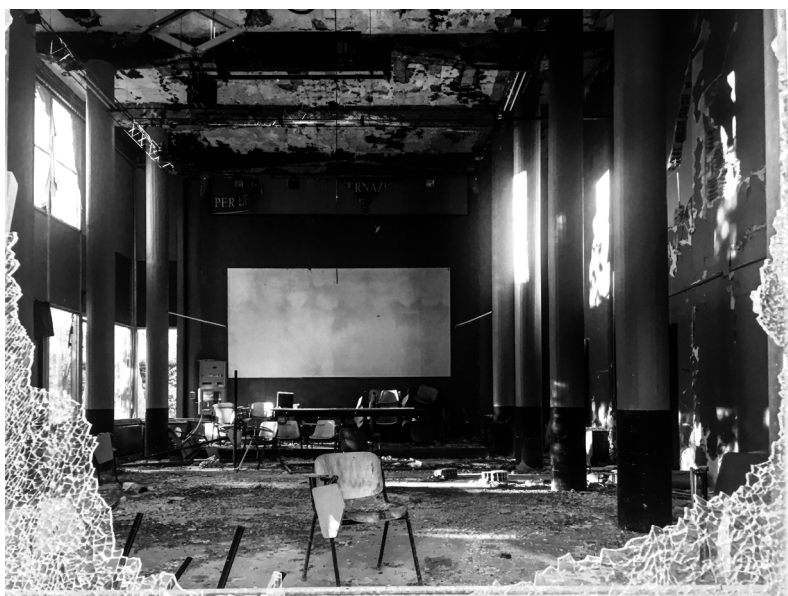
Figure 14.5 Ruined building. Photo: Fatima Marchini.
