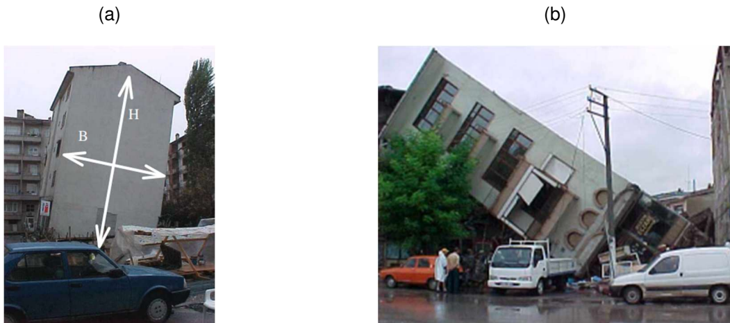
Figure 1. Examples of damages in Adapazari after the 1999 earthquake: (a) vertical displacements with significant tilt ( H/B=1.7 ) and (b) bearing capacity failure ( H/B=3.2 ) (modified after Sancio et al. 2004).
