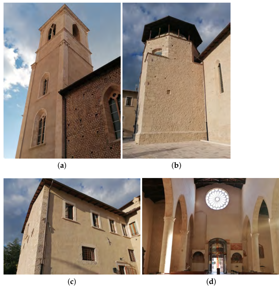
Figure 4. The St.Silvestro complex after the rehabilitation works following the 2009 earthquake: (a) Belfry, (b) Chapel, (c) Canonical house, (d) Interior of the church.
